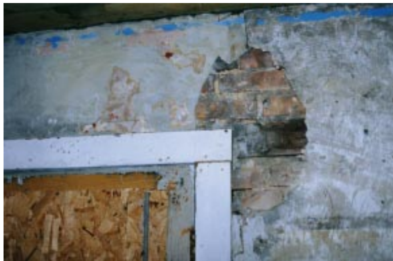
Fig. 3. A single hand-hewn lintel stretches across each door and window combination in the east room addition.
