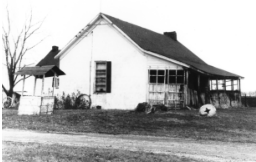
Fig.1. The Five Mile House sometime in the early 20 th Century sported an enclosed porch and a probably fake well. Note also the kitchen ell with its gable end chimney.
