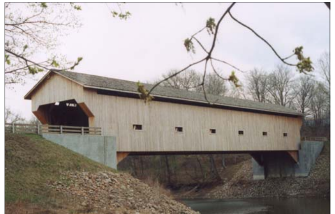
Designated as the longest, clear span, wooden covered bridge without a load restriction in the United States, this scenic, covered bridge sits astride the Embarras River just west of Greenup, IL.
