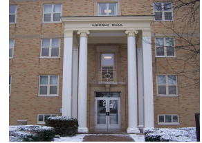
Lincoln Hall—North Doors
