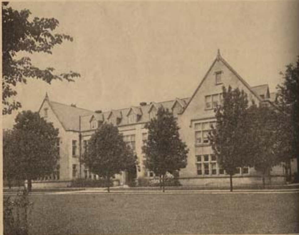
THE TRAINING SCHOOL BUILDING
